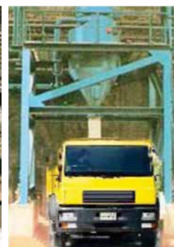
Intercept cyclonic hopper discharging on truck for disposal.
