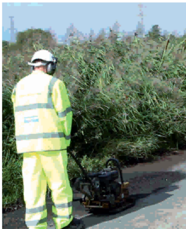
Cleaning and compaction with the help of plate compactor
