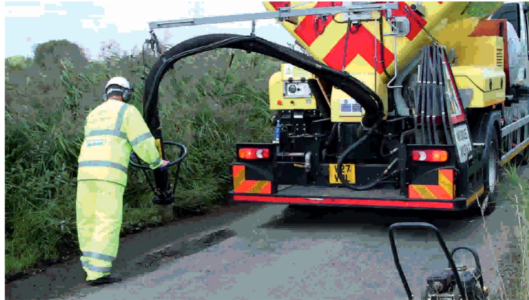
High velocity air is used to remove all dust and debris from the surface leaving a perfect base for repairs.
